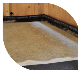
Laying of acoustic mats
